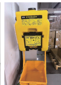
Installing eyewash stations
