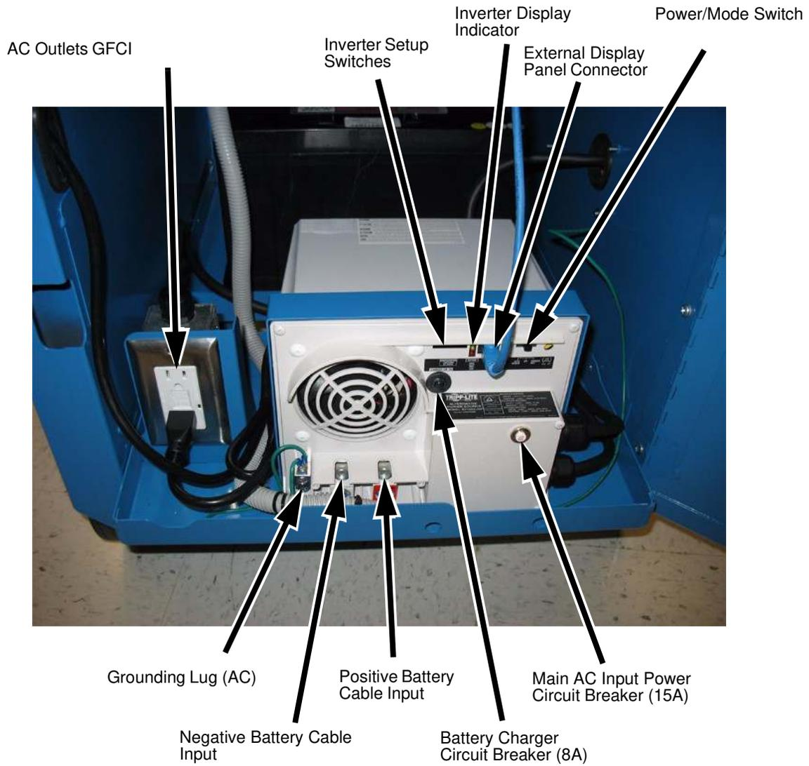
**Figure 8. Power Module (Inverter/Charger) Features and Safety Devices
